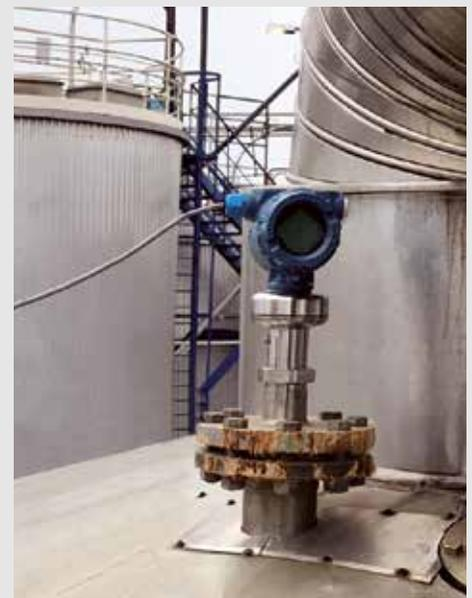
*“The Rosemount 5408 was able to handle turbulence, foam, and agitators and provide a reliable, stable level measurement.”*
